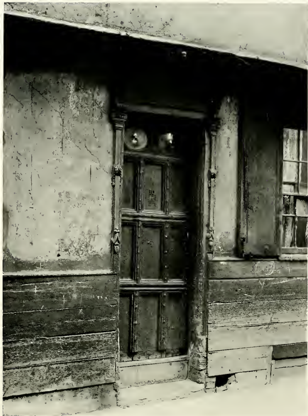
DOORWAY DETAIL OLD HOUSE AT IPSWICH The oval lights of English crown glass admit light into a small hall
